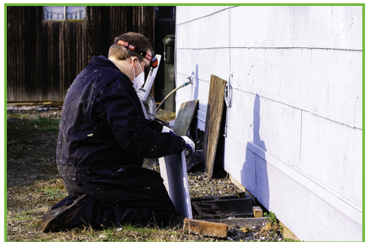
YCAP's lead Energy Services Technician conducts a home weatherization inspection.
